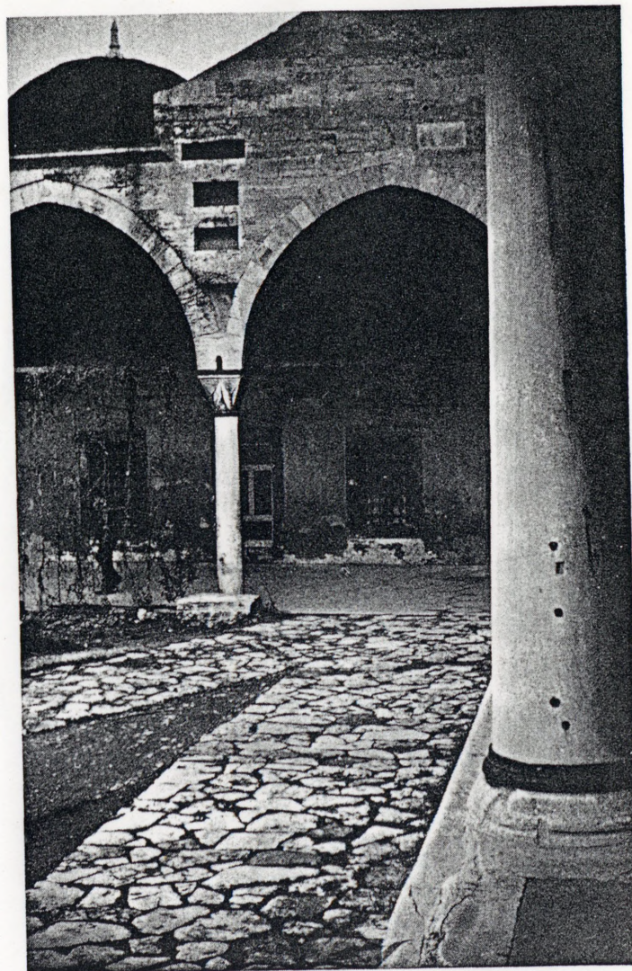
Istanbul. Edirnekapi. The Mosque of Mihrimah. Reused Byzantine Proconessian columns, one clearly showing the holes to which crosses and icons were fixed.
