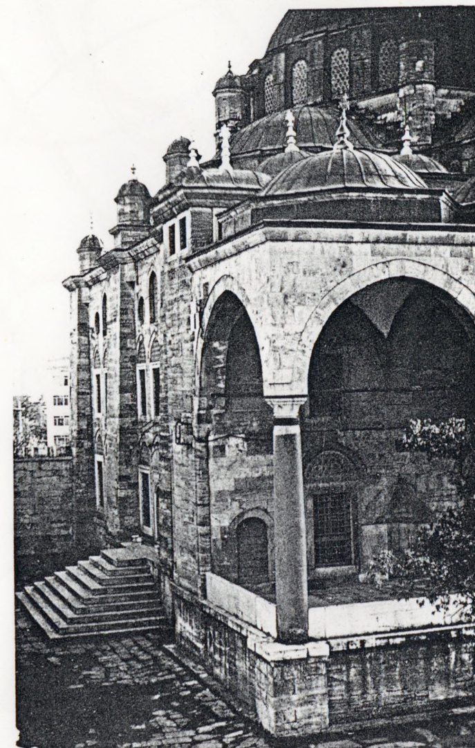
Istanbul. The Mosque of Hekimoğlu Ali Pasha, showing a reused Byzantine granite column cut roughly at the neck to fit the capital.
