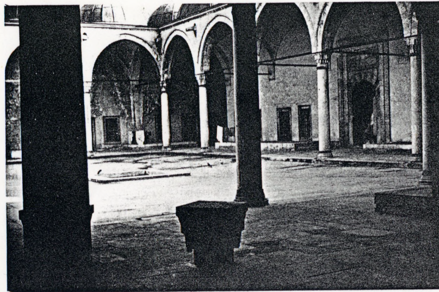
Istanbul. Süleymaniye Complex. Tabhane Courtyard with reused Proconnesian columns. The capital in the foreground is in the process of carving.
